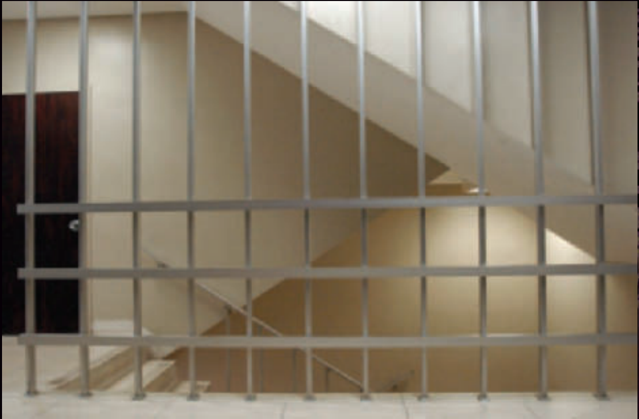
Another example of geometric design: the staircase is accented with a metal rendition of the building's exterior concrete screening.
