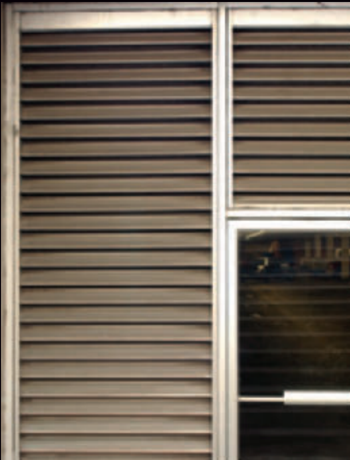
Only from the below ground entrance (screened horizontally in keeping with the courthouse's facade) is the parking garage visible. ★
